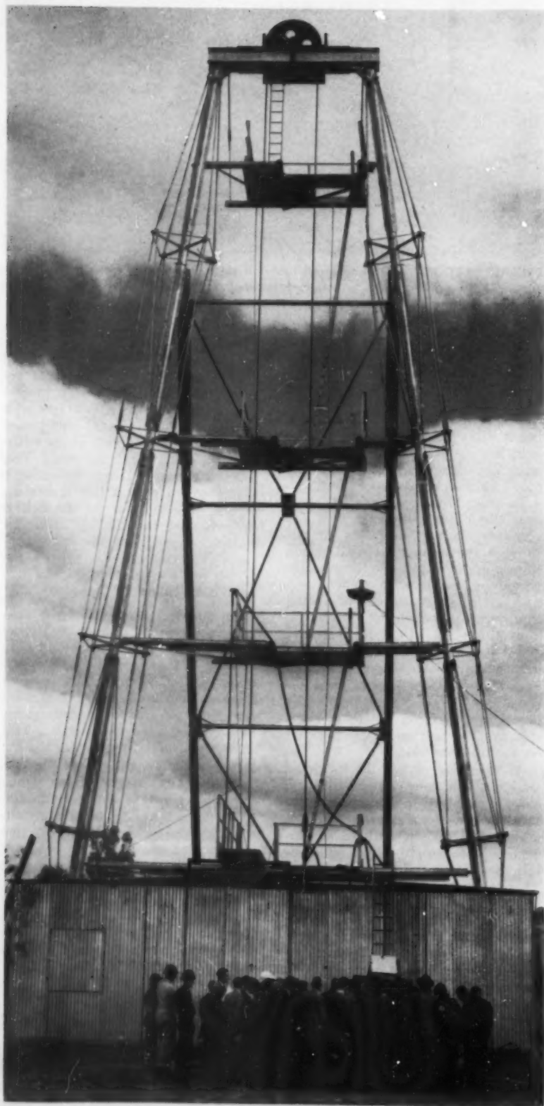
DEEP DRILLING at North Broken Hill Limited is inspected by convention delegates. Note the special trussing on the derrick legs. Sixty foot pulls are routine.
